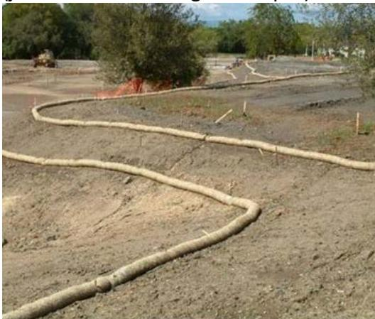
On long bare slopes, place a series of wattles. If it's nearly flat, space wattles every 20 feet. For steep slopes (2:1), space them every 10'. For moderate slopes, every 15' is fine. **Extremely steep slopes** don't benefit from wattles. Instead of trying to stop the flow halfway down a steep slope, try to stop it up top on the ridge.
